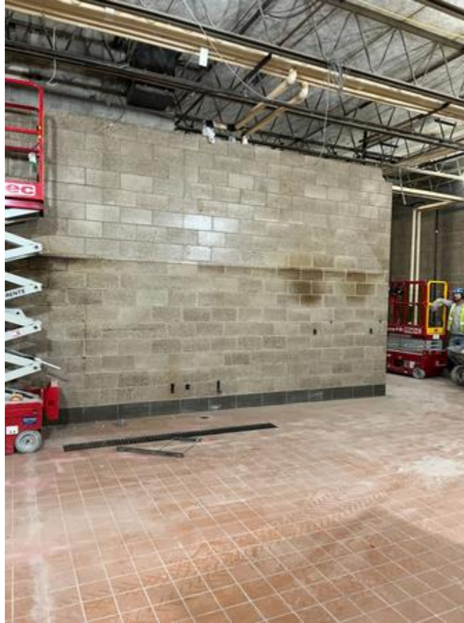
Demolition of kitchen and cafeteria area ongoing
