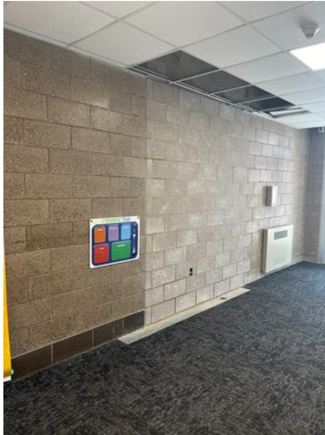
Block infilled at main entrance
