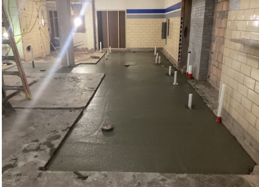
New concrete floor infills in boys' locker room.
