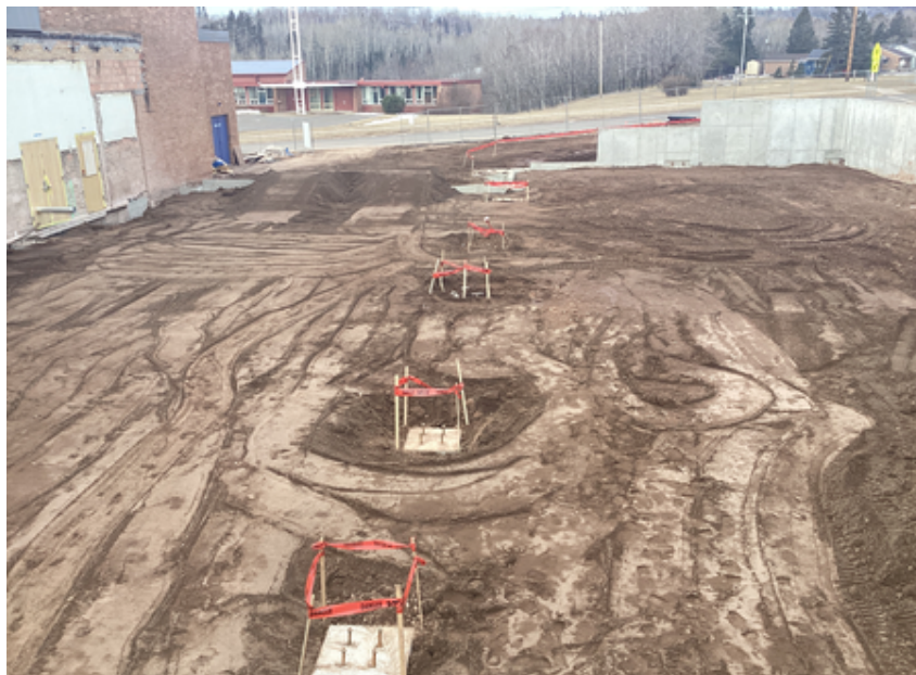
Backfill and soil grading/compaction Area B Music Suite
