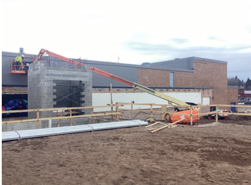
Metal panel reinstallation Area B Music Suite
