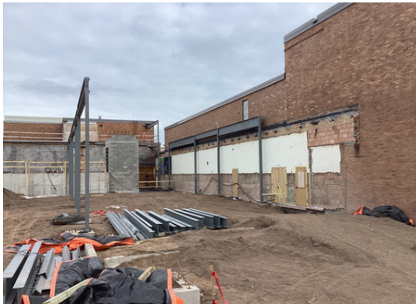
Structural steel installation Area B Music Suite
