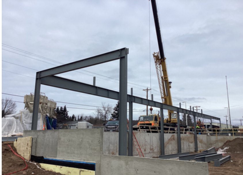
Structural steel installation Area B Music Suite
