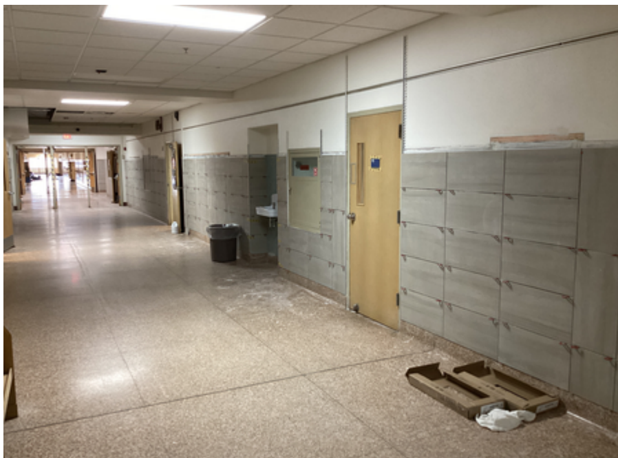
tile work in corridors.
