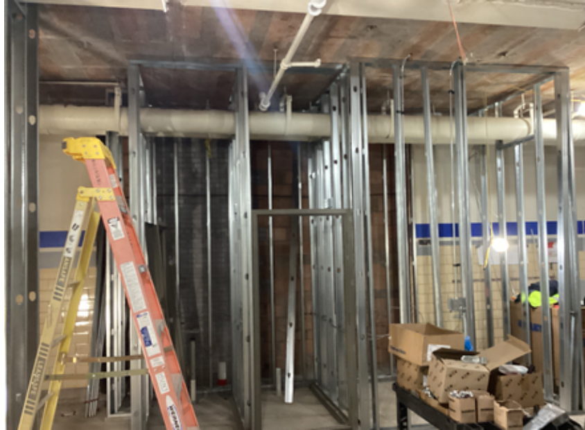
Wall framing and electrical rough ins in boys' locker room
