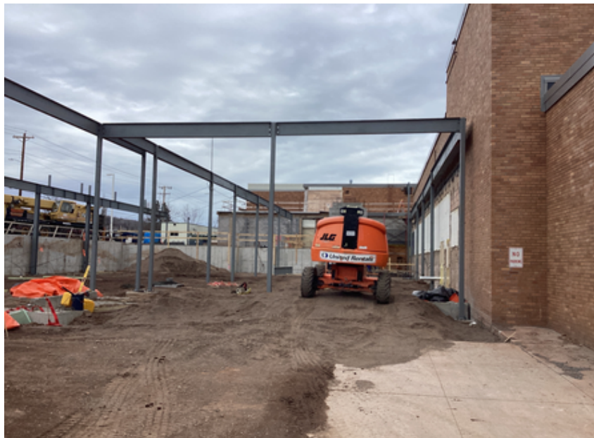
Structural steel installation Area B Music Suite
