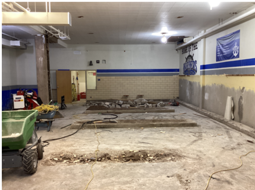
Demolition in girls' locker room
