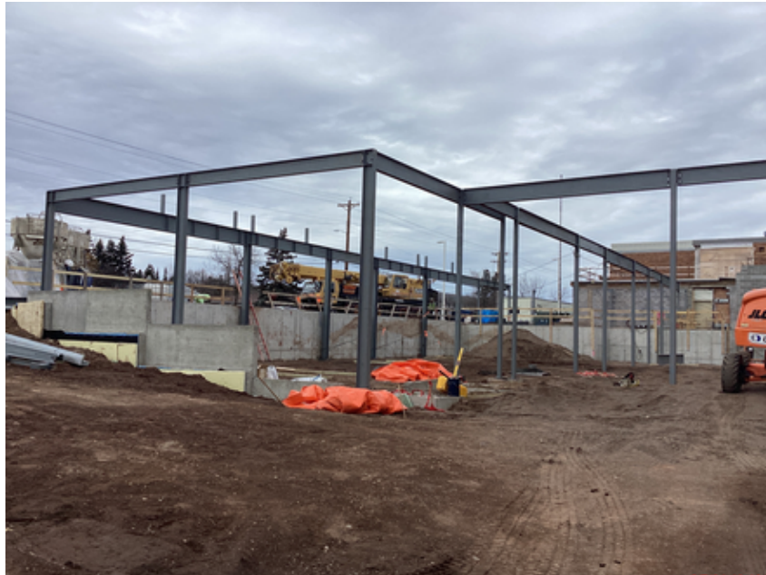
Structural steel installation Area B Music Suite
