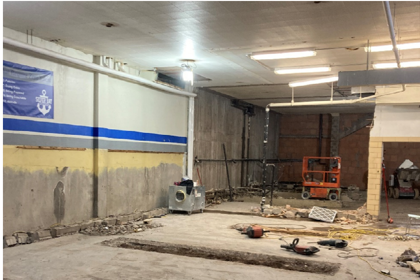
Demolition in girls' locker room
