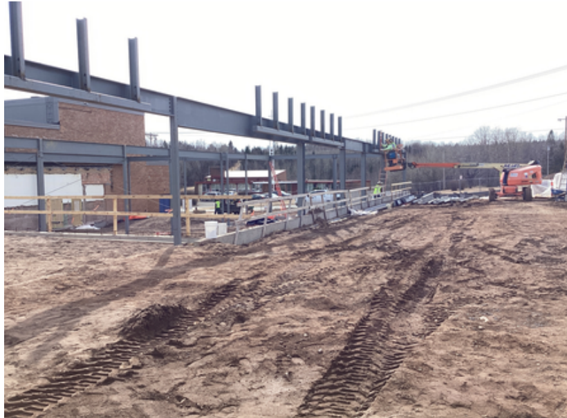
Structural steel installation finished at Area B Music Suite
