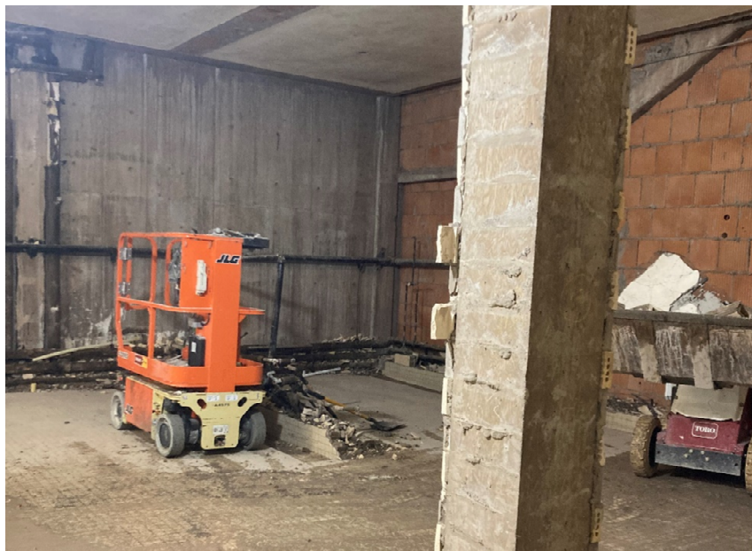
Demolition in girls' locker room
