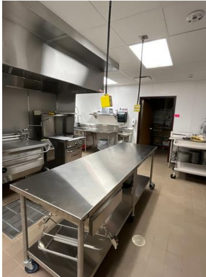
Kitchen completed. Staff moved-in and starting using new space
