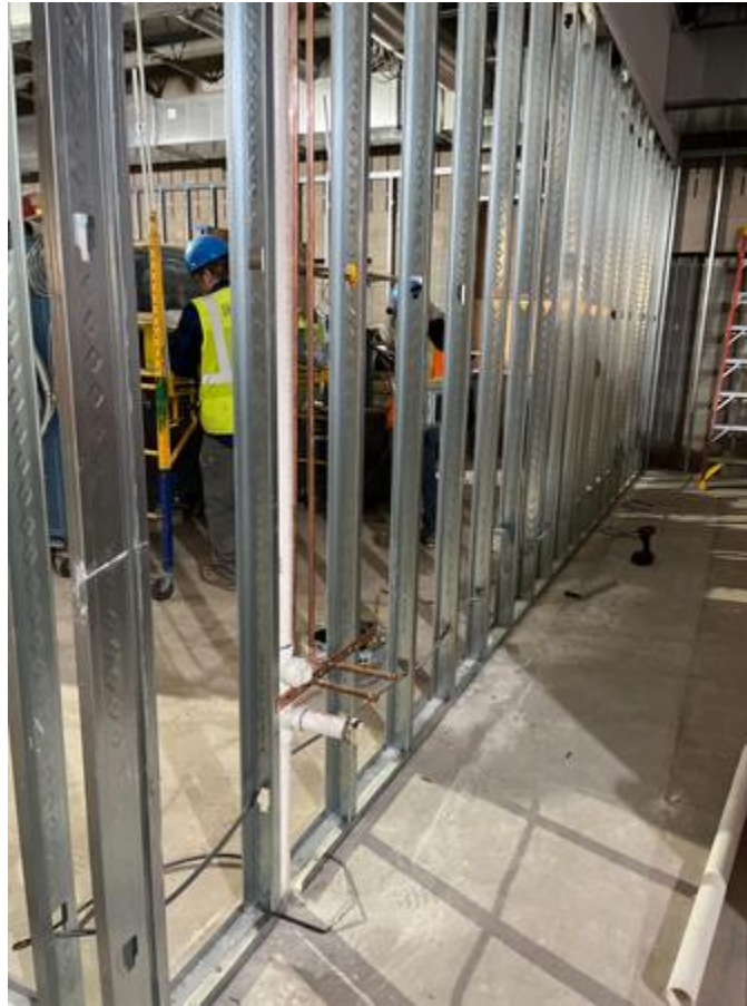
Steel stud framing and rough-ins ongoing
