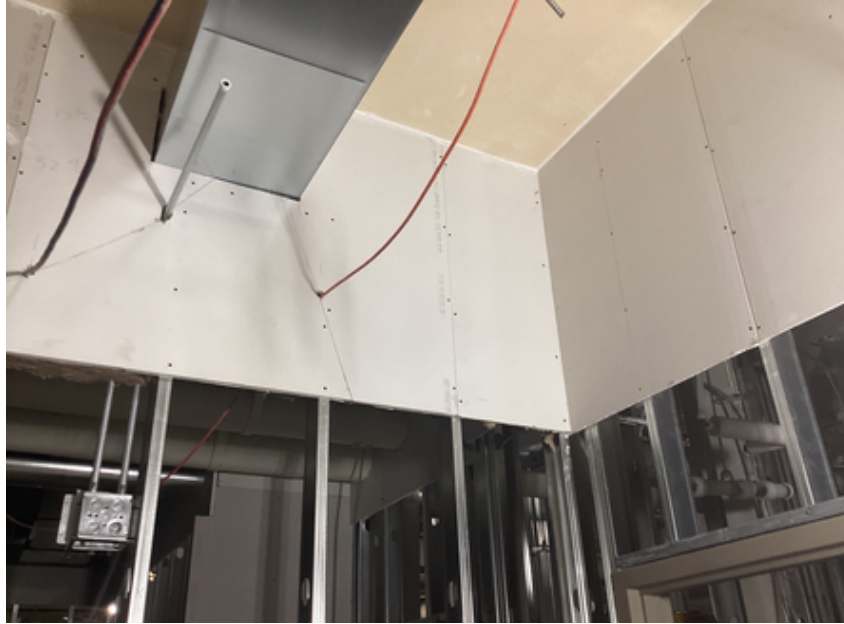
Drywall work in boys' locker room
