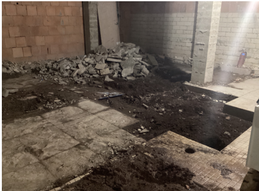
Floor removal in girls' locker room
