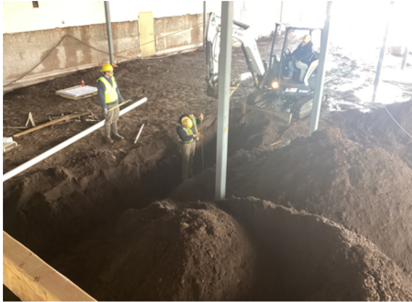
Underground plumbing at Area B Music Suite
