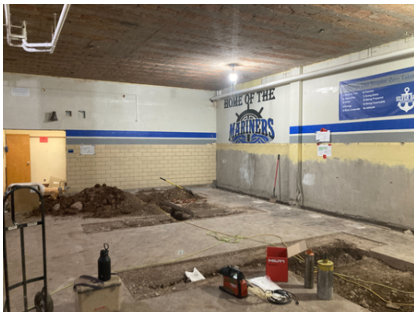
Floor Demo at Girls' Locker Room
