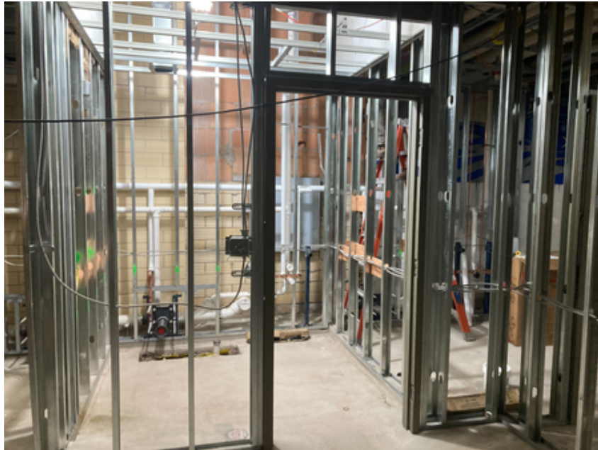
Plumbing and electrical rough in in boys' locker room
