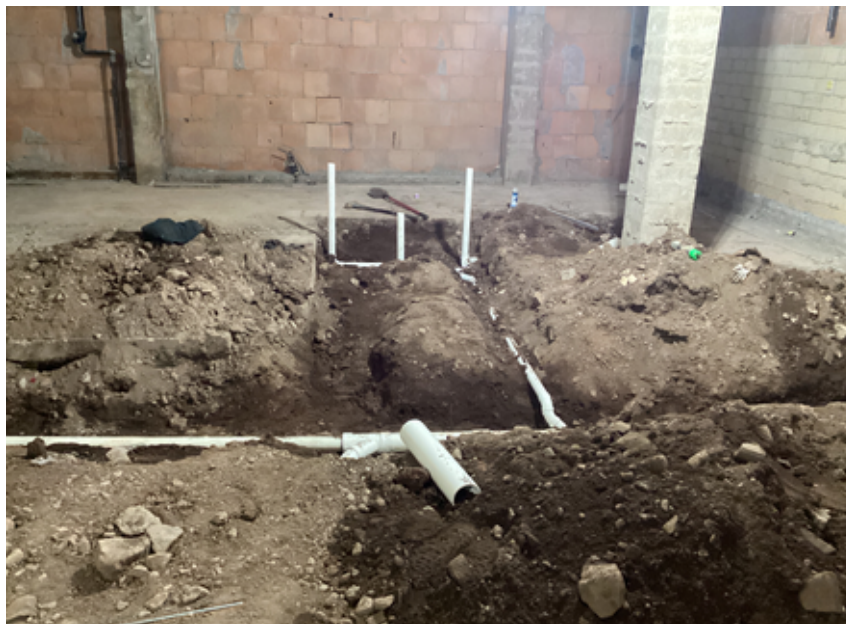
Underground plumbing at Girls' Locker Room
