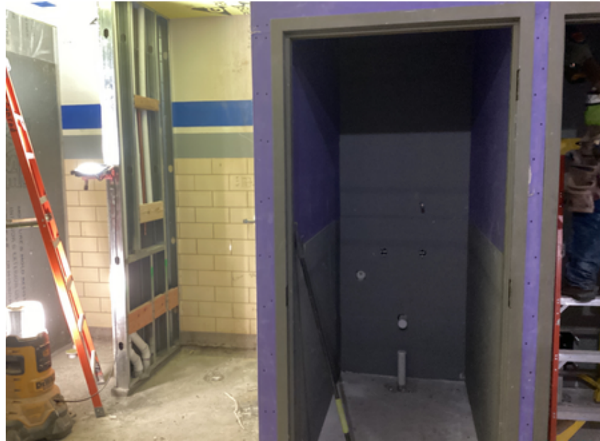
Cement board walls in boys' locker room
