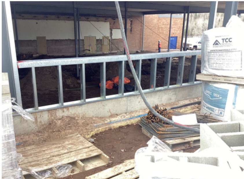
Exterior wall framing at Area B Music Suite
