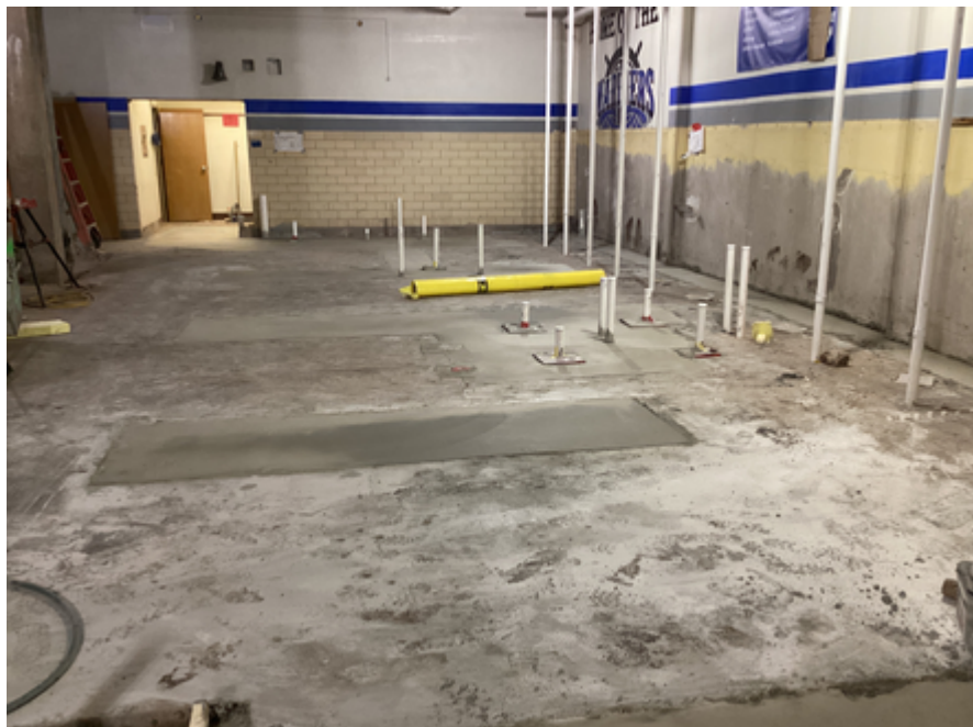
Underground plumbing and floors poured back at girls' Locker Room
