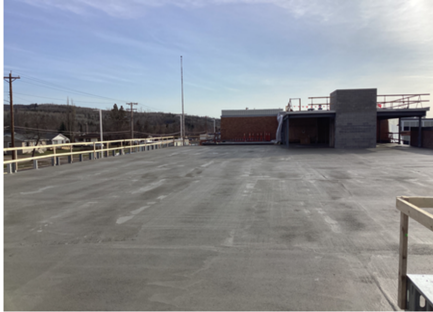
Precast plank concrete topping at Area B Music Suite
