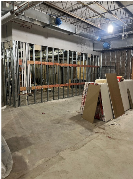
HVAC Ductwork Rough-Ins finishing up. Topping out sheetrock.
