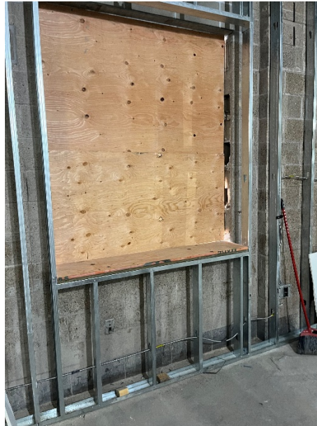
Steel stud framing at window openings
