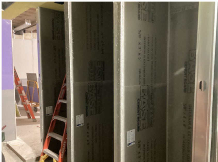
Cement board and gyp board walls in boys' locker room
