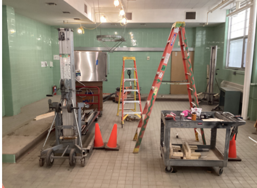
Demolition in kitchen
