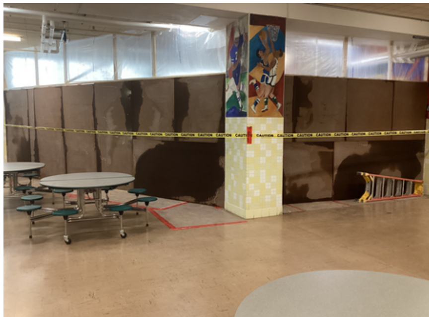
Temporary construction wall between cafeteria and kitchen
